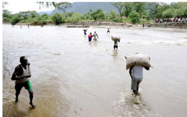
Residents assist in carrying people and goods across the Weiwei river in West Pokot County. Weiwei bridge was damaged by floods. Sebit bridge was also washed away cutting off transport between Kitale and Lodwar. [Kevin Tunoi, Standard]
